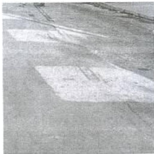
Exhibit 27. A tire skidding across an irregular area, such as a pavement patch or chuck hole, may bounce
