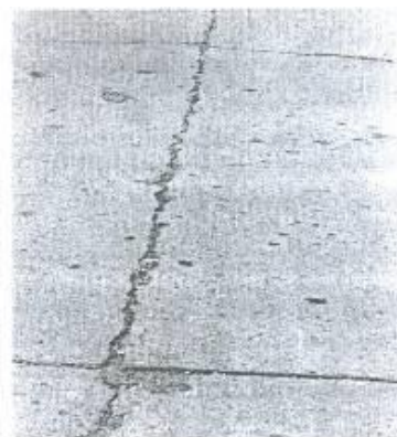
Exhibit 4. On Portland-cement concrete, skidmarks may be nearly invisible.
